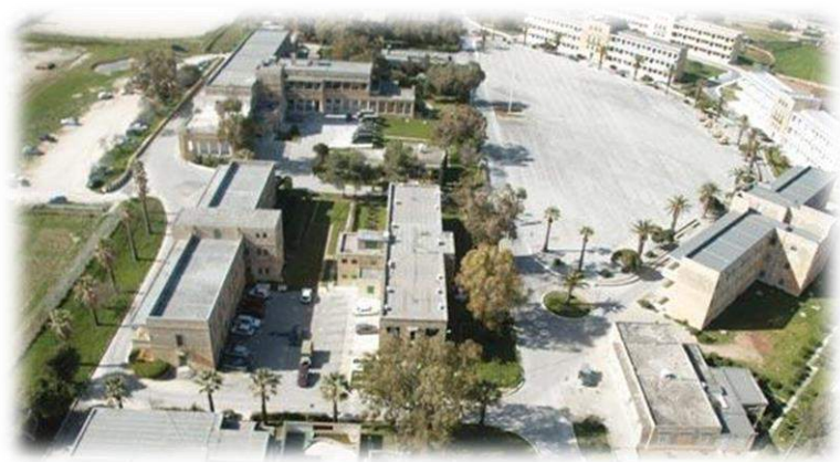
Figure 14: Ex-Malta International Airport at Luqa
